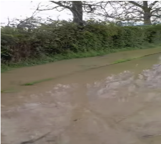
Photo 1:- Canal overtopping at Bridge 88
